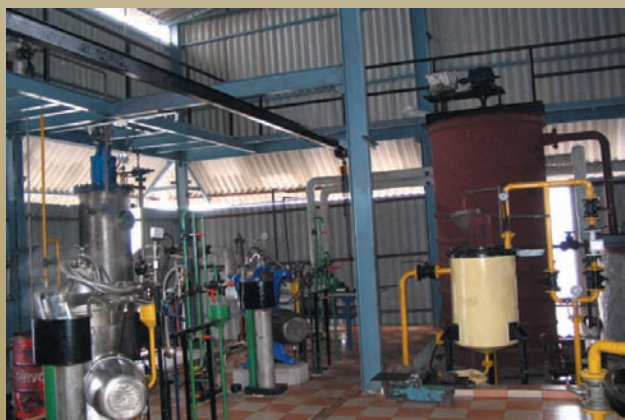
Enzymatic Degumming Section of a Refinery
